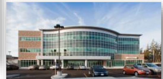
Springbank Medical Centre London, ON
